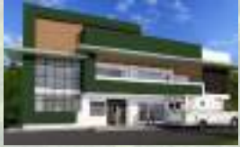
Construction of ₱12 million Infirmary Building in the Main Campus.
